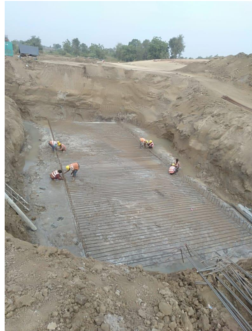
MJB Steel winding A1 LHS at Ch 359+936
