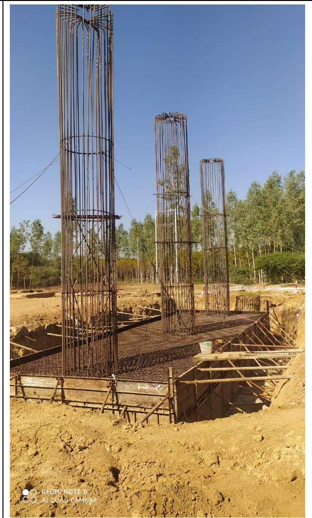
Pile Cap Steel at MJB 351+282
