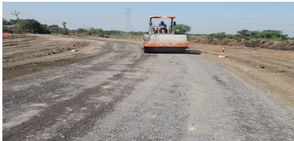
Diversion Rolling at ch. 362+000
