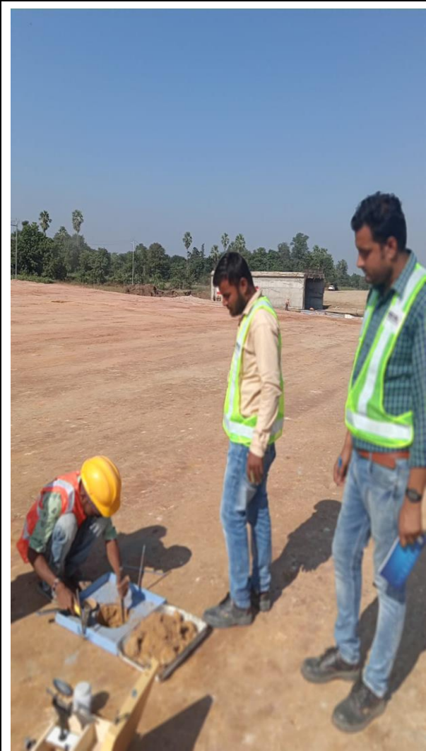
Embankment FDD checking at Site
