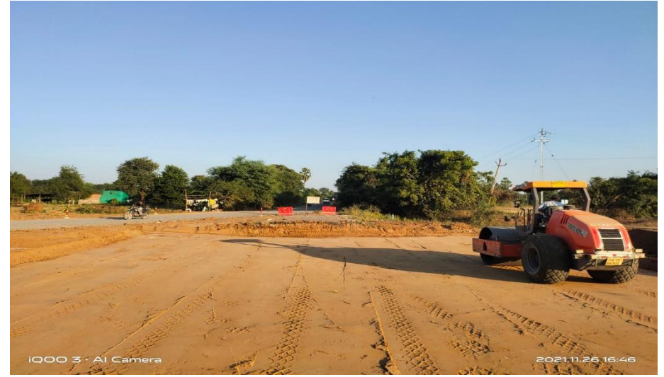
LVUP Bed Compaction @ 356+849 LHS
