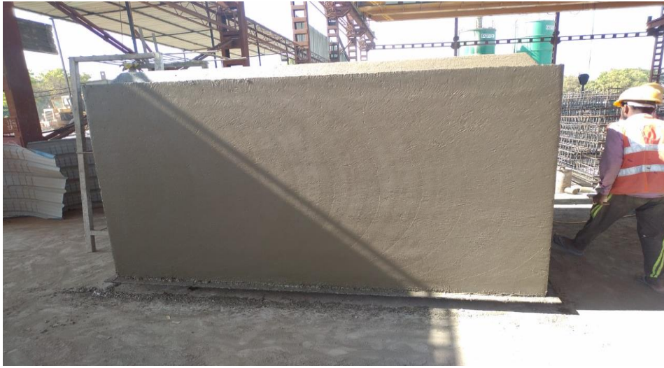
Pre Cast Box Culvert Segment Casting at Plant
