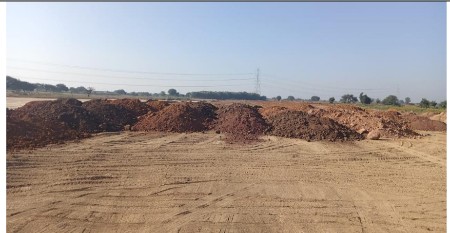
Dumping of Embankment
