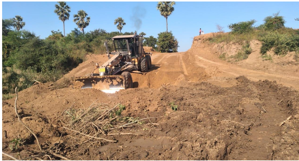
Approach work in progress @358+100 A-1 side
