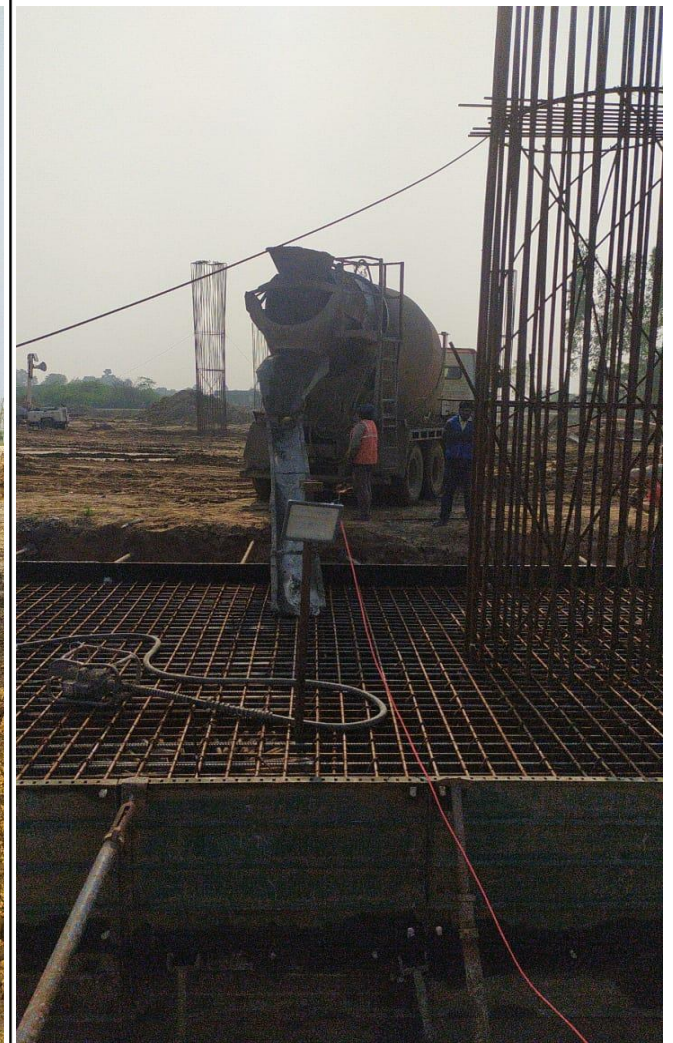
Pile Cap Pouring at ch.352+281 MJB
