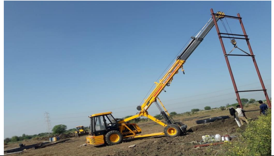
Electrical DP pole erection
