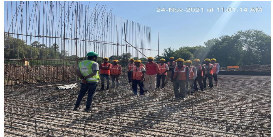
Safety - Tool Box talk in A1 site at site
