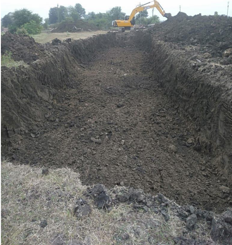
Box Culvert Excavation at ch.367+650
